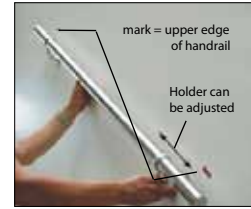
Fasten stair bolt
