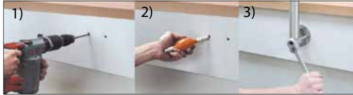
1) boring 10ø 2) blowing out 3) Bolt (without dowels) with concrete screws B37
