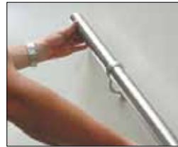
Put handrail in bracket
